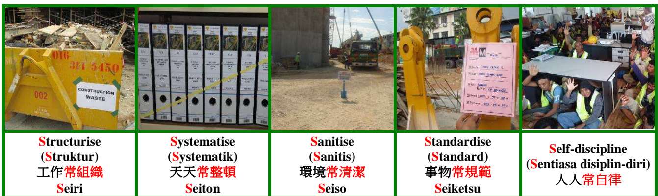
Fig-1: typical examples of 5-S implementation at construction sites (5 out of 50-points)
